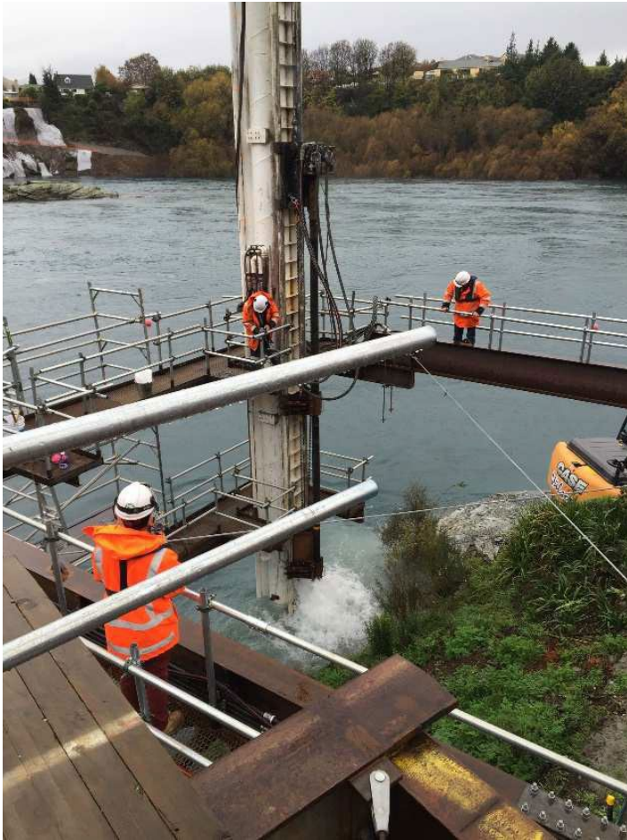
Spotters inspecting the drilling rig in operation
