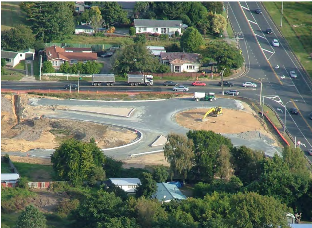
Gordonton Road – SH1 Roundabout Intersection
