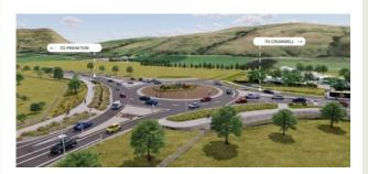
The Howards Drive roundabout will make this intersection safer. Safety concerns have seen this T-intersection prioritised because the speed through this area is higher and is currently controlled by a give way sign. The roundabout will be similar to those at Stalker Road, Hawthorne Drive and Grant Road. Better access to the Ladies Mile Pet Lodge will be provided from the north side of the roundabout.
