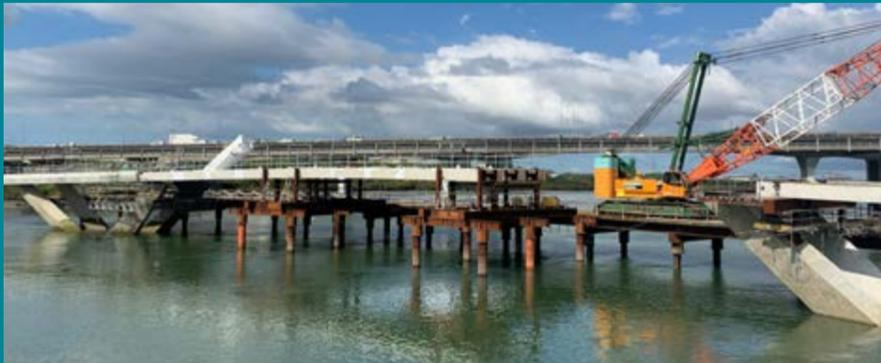
The temporary platforms to support the steel central deck
