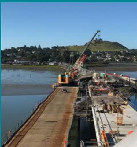
Looking south towards Māngere Bridge. Above the arch, the temporary working platform on the left and the new bridge deck under construction.
