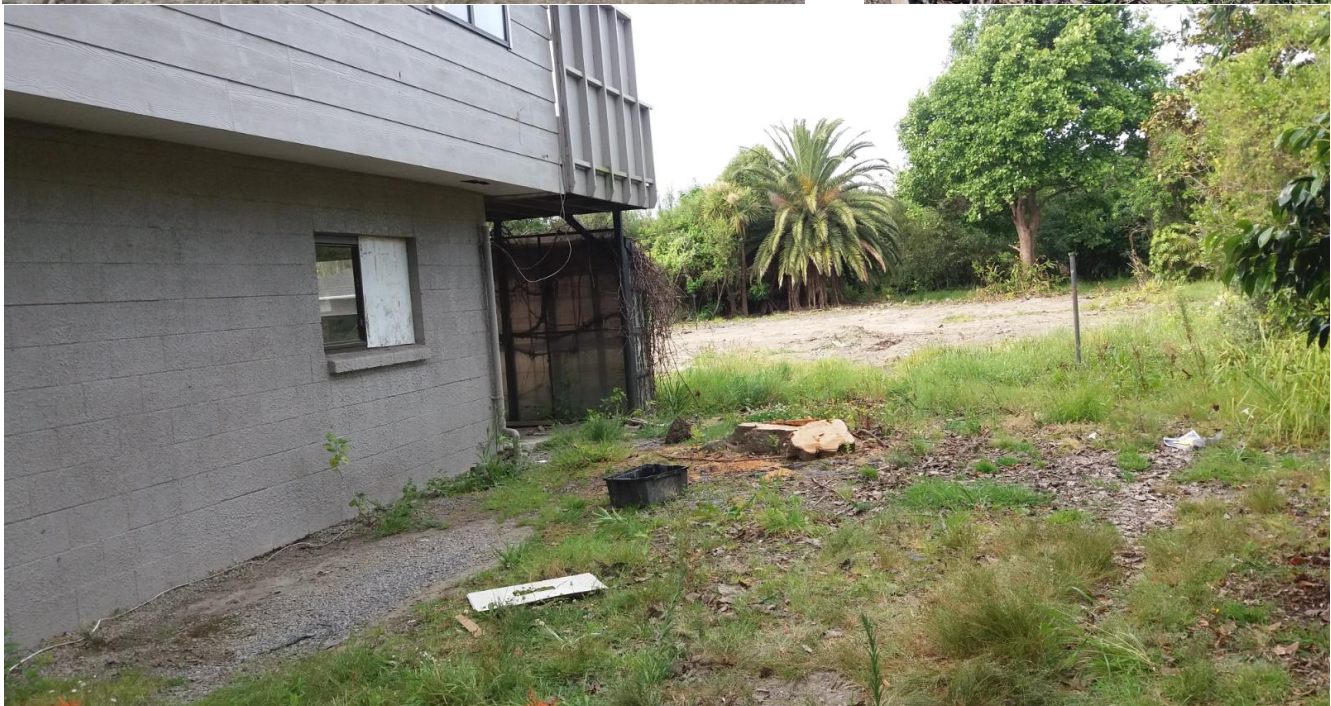
Vacant residential buildings with surrounding topsoil and vegetation (photos taken: November 2017)
