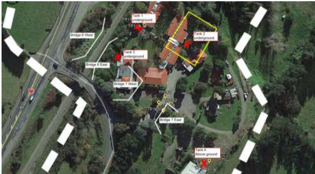
Figure 3: Location of the four storage tanks marked in red on the Bridge Lodge site.
