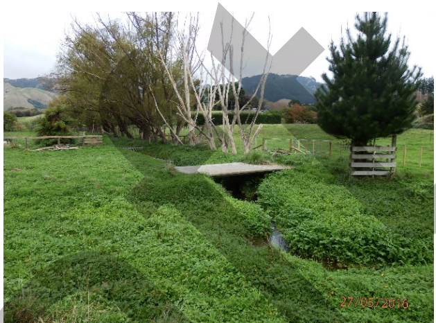
Fig. 2 Main crossing and existing gate on true left Bank.
