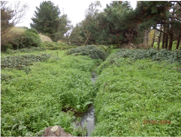
Fig. 5 Stream channel at northern foot bridge, looking downstream: note blackberry.
