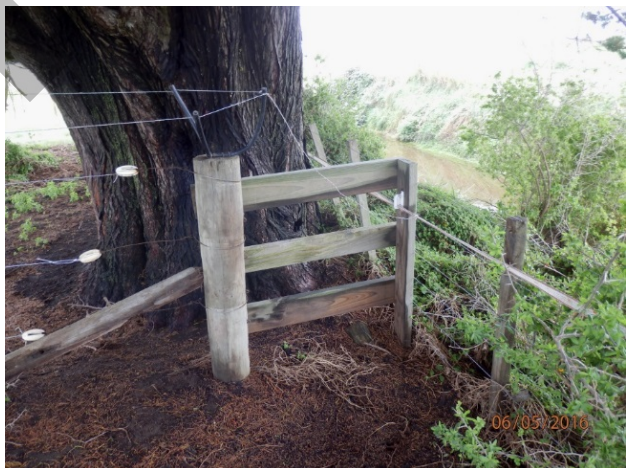
Fig. 4. Rails connecting side fence.
