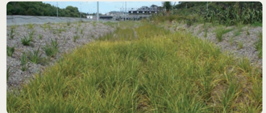
Example of a vegetated swale
