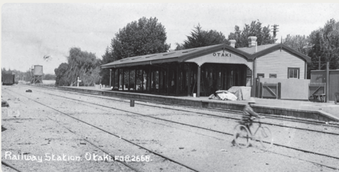
Ōtaki Railway Station by Frederick George, 1863-1923 Radcliffe (photographer) ca February/March 1911
