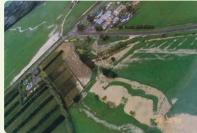
Existing State Highway 1 and North Island Main Trunk Railway crossings of Mangaone Stream at Te Horo following 28 October 1998 flood (photo courtesy of Greater Wellington Regional Council)
