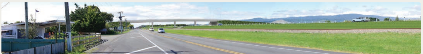
View looking north on existing state highway - indicative mitigation shown
