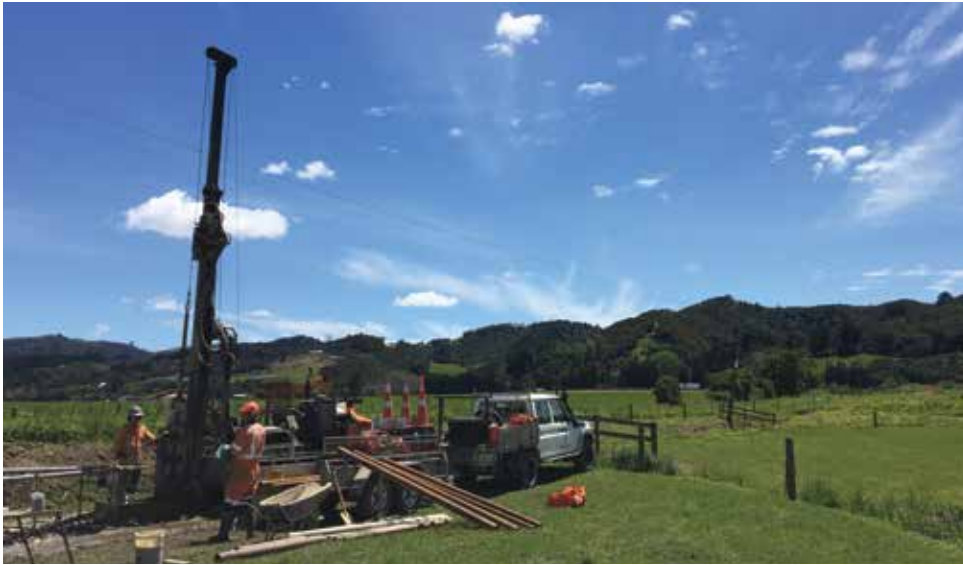
Geotechnical work on the proposed new route of SH2
