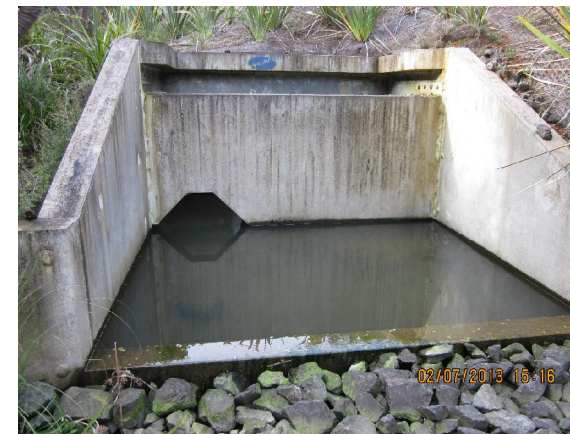
TYPICAL IMPACT BASIN (FROM NORTHERN GATEWAY TOLL ROAD)
