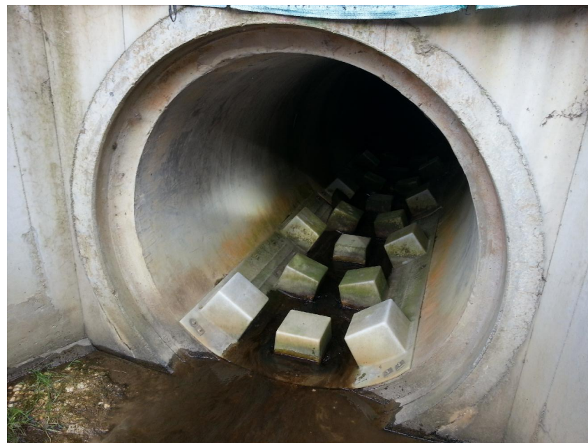
TYPICAL FISH PASSAGE BAFFLES (FROM NORTHERN GATEWAY TOLL ROAD)
