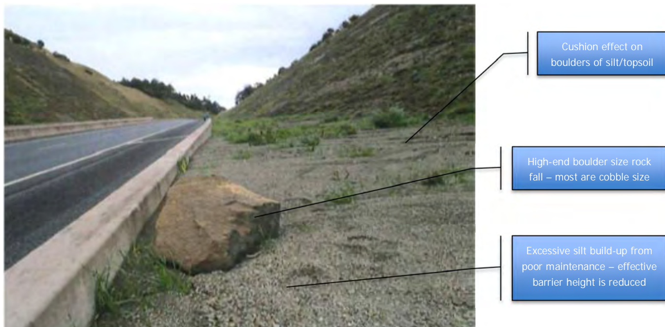
Figure 13: Example of rock fall contained by rock fall ditch and barrier protection design on NGTR.
