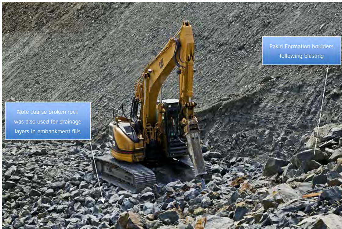
Figure 19: Breaking of Slightly Weathered Pakiri Formation rock following production blasting (NGTR construction, NGA).
