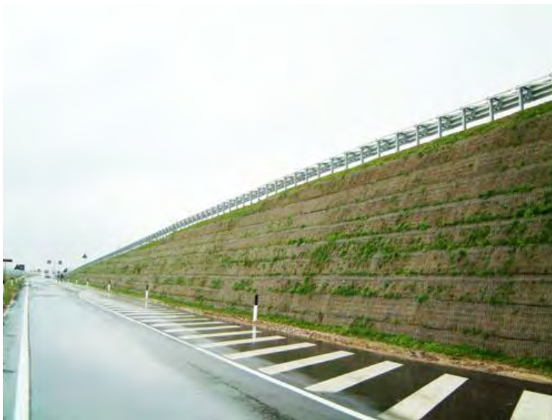
Figure 16: Example of MSE slope with vegetation under establishment using wrap around geogrid.
