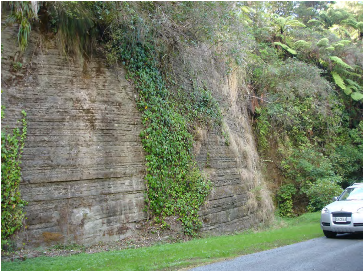
Figure 6: Closely bedded weak alternating sandstone and siltstone in the Perry Road area.
