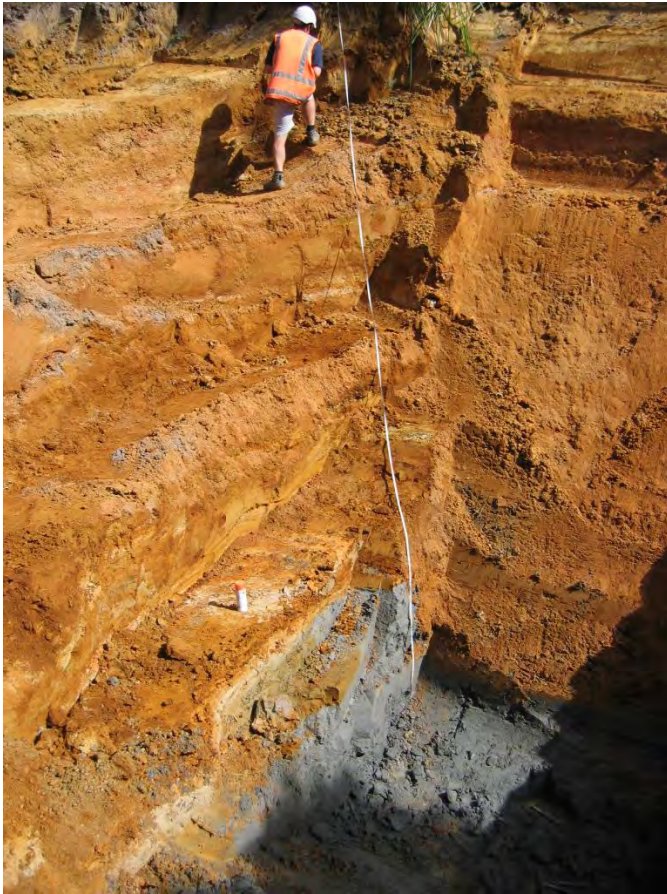
Figure 14: Excavation to beneath weathering zone for shear key on Northern Gateway Toll Road project
