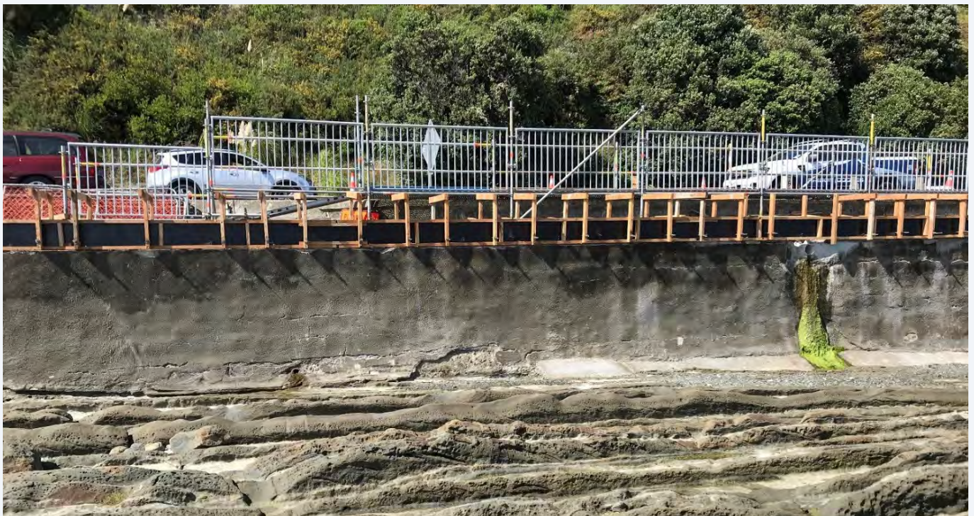
Boxing ready for concrete to be poured as part of the seawall repairs at Magazine Point.
