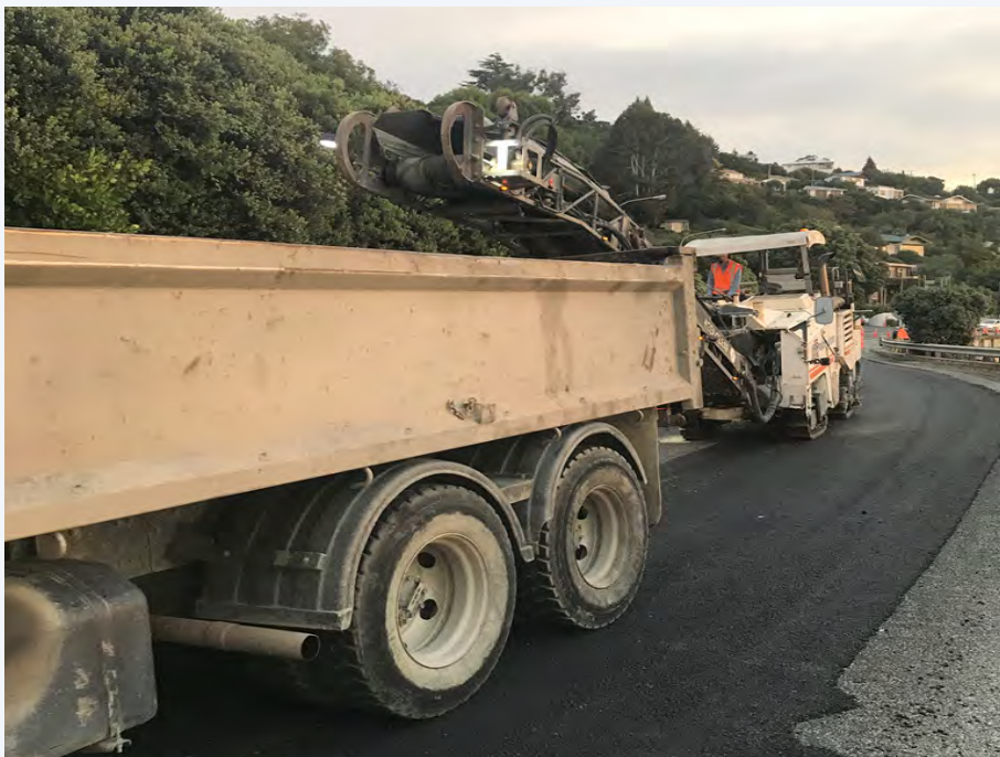
The milling machine in action, feeding out cut material into the truck.
