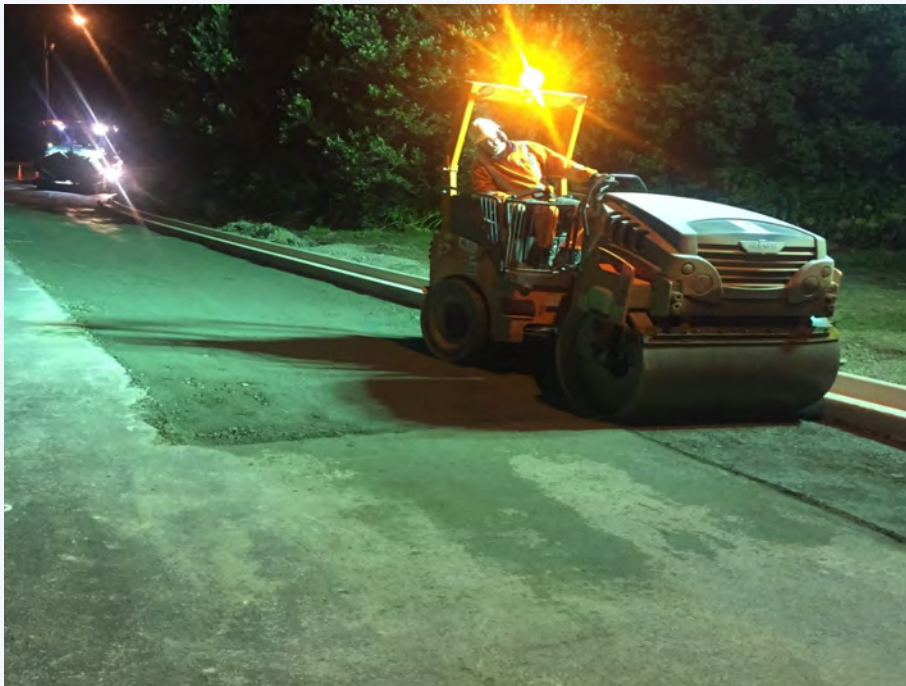
Completion of the dig out of soft area at Magazine Point.
