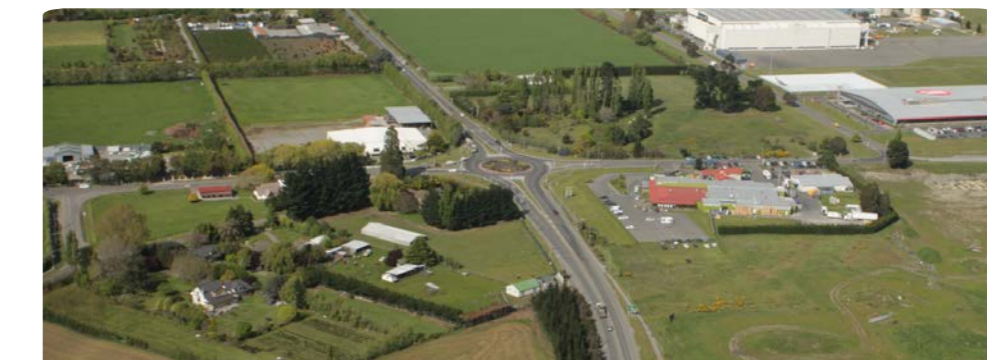
Harewood Road roundabout
