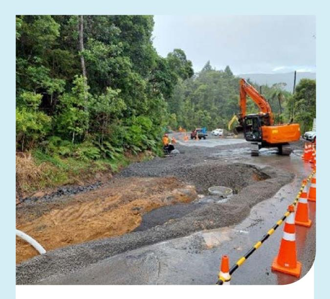
Effective stormwater and sediment management plays a major role in protecting the environment through construction. We're installing silt fencing, rainwater capture drains and sediment tanks to ensure any stormwater runoff is collected, diverted, and treated before it reaches the local waterways.
