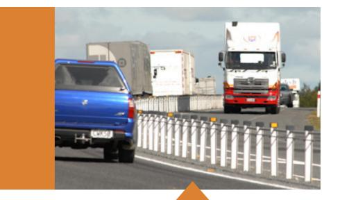
something less forgiving like a tree or another vehicle. The wire cables flex on impact, slowing the vehicle and pushing it back into its lane.
