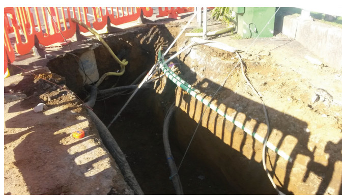
Some of the existing services near Mangorei Road intersection.
