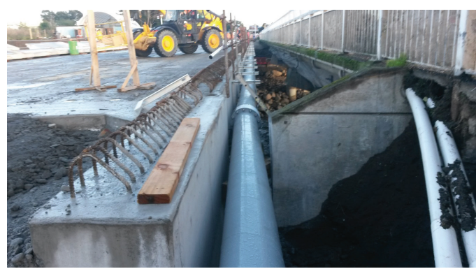
The new water main being installed on the new Waiwhakaiho Bridge.
