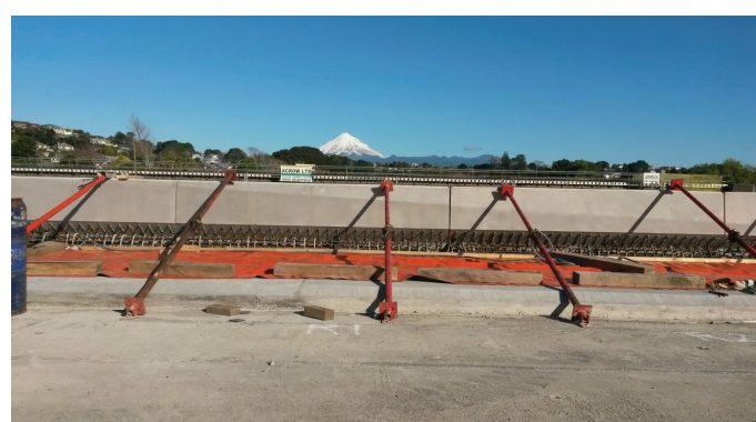
Concrete safety barriers being installed on the new Waiwhakaiho Bridge.
