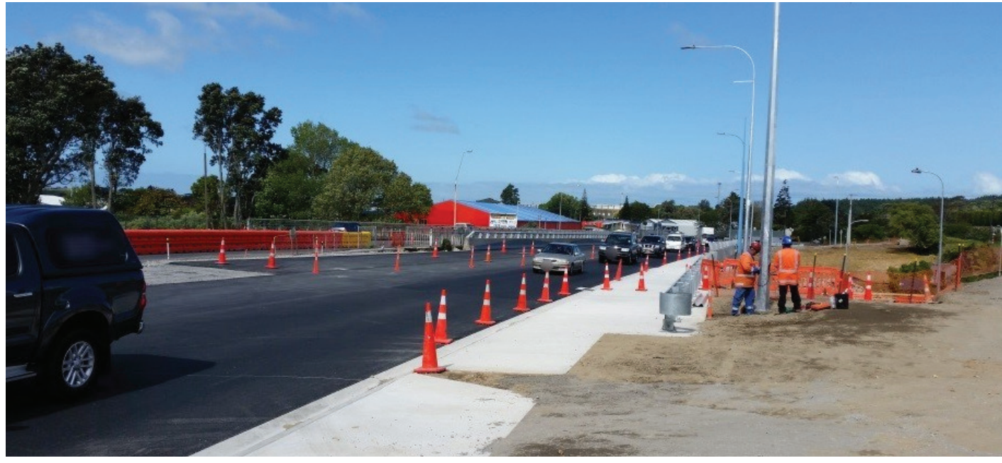
Vehicles driving over the new Waiwhakaiho Bridge
