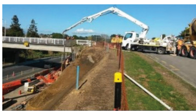
Pumping concrete at Paynters Ave
