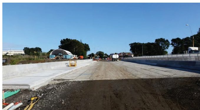
We've almost finished the new Waiwhakaiho Bridge!
