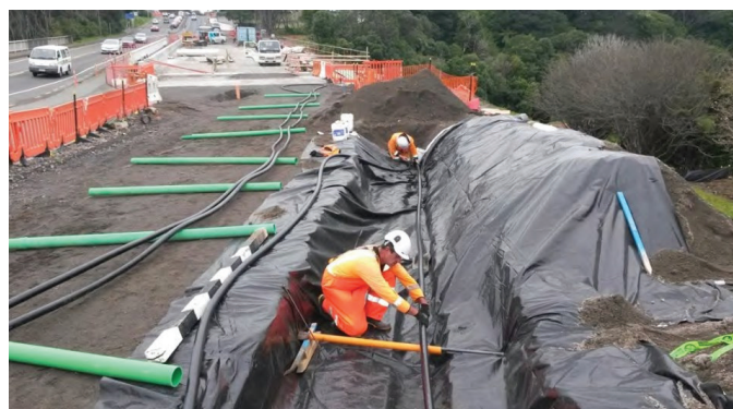
Pulling power cables across the new Te Henui Bridge.
