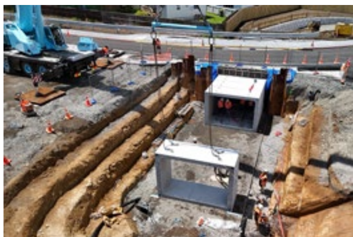
Concrete frame being installed for the underpass
