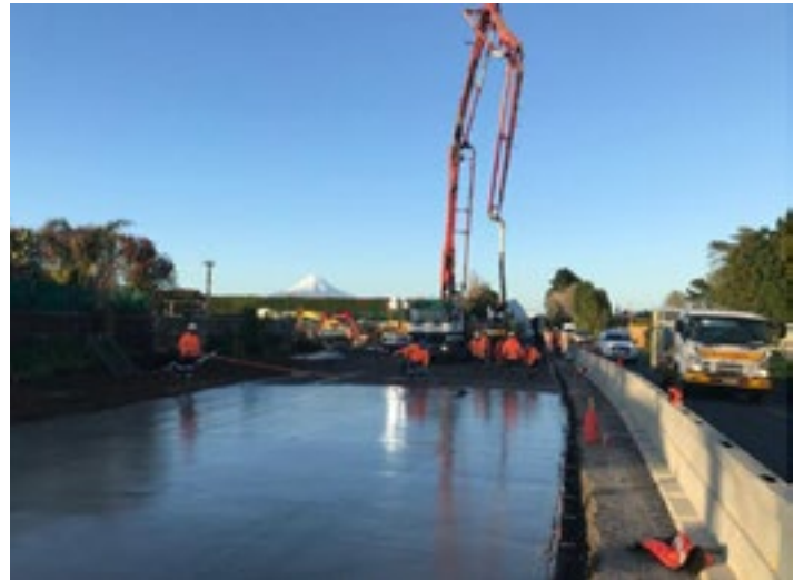
Pavement work being completed on the state highway
