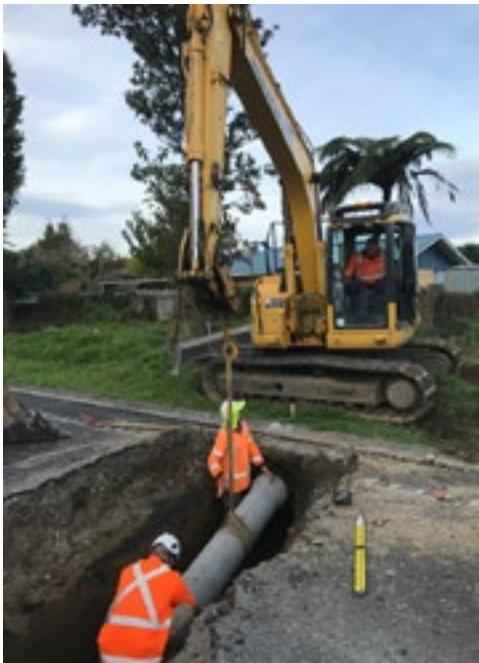
Installing a pipe to handle stormwater
