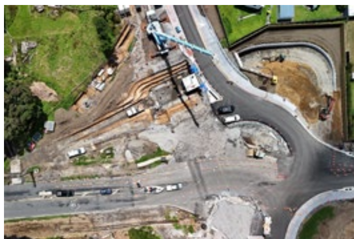
Aerial view of the underpass under construction
