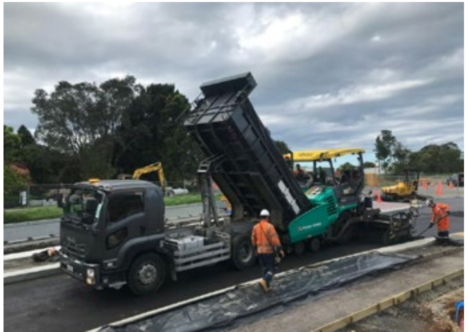
Laying asphalt on the highway
