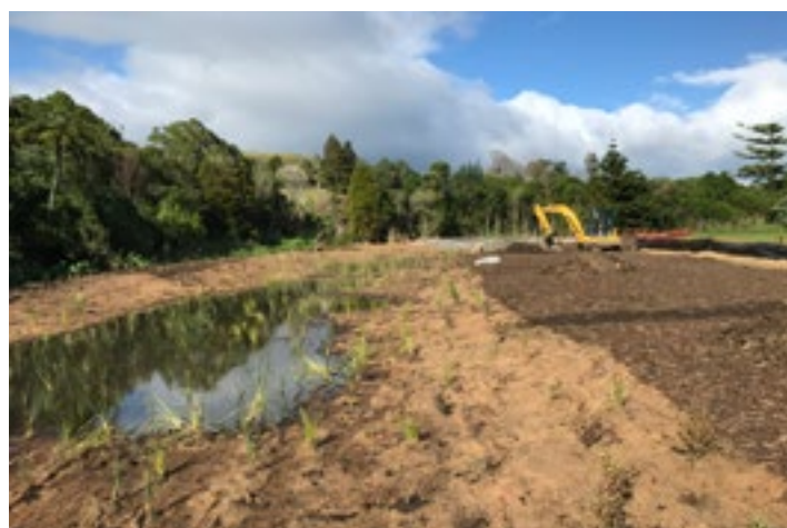
Construction underway on the stormwater wetland swale
