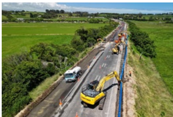
Completing work on the highway during the summer closure
