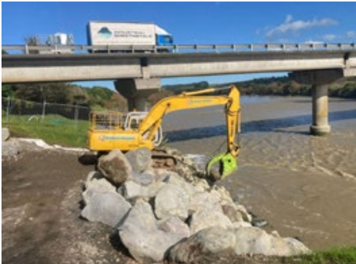
Placing rip rap for the stormwater outfall at the Waitara River
