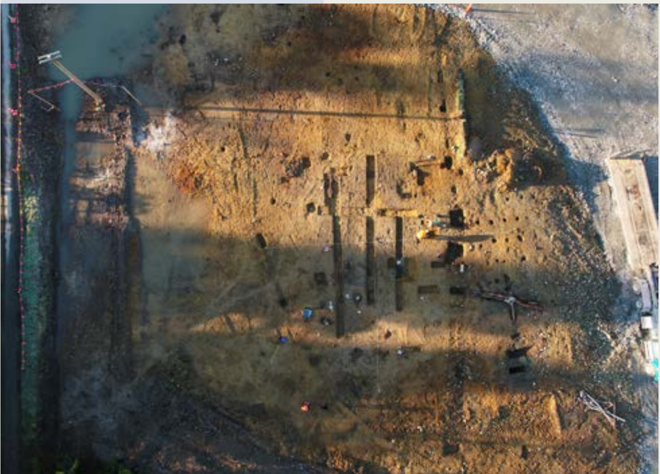
Aerial view of the old presbytery building site.
