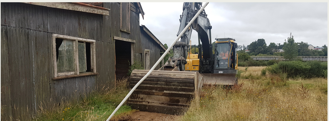
A digger strips back topsoil alongside Gough's stables.
