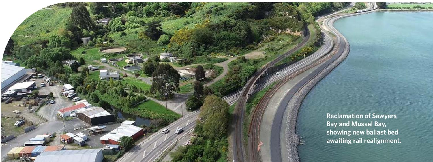
Reclamation of Sawyers Bay and Mussel Bay, showing new ballast bed awaiting rail realignment.
