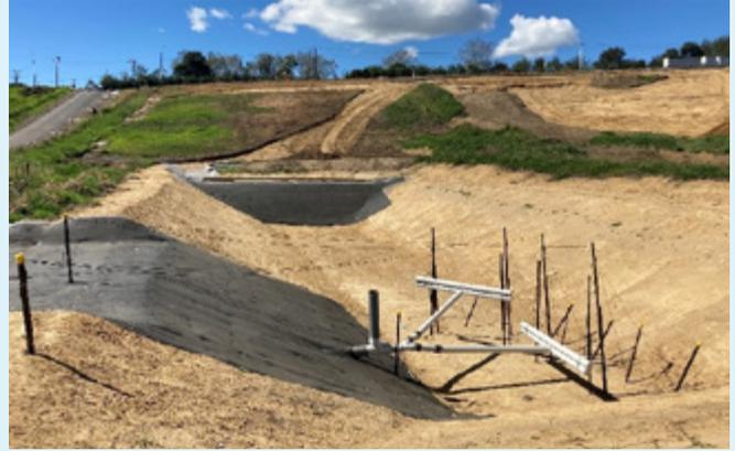
Sediment retention pond located next to Harrison Road can hold 540m<sub>3</sub>.
