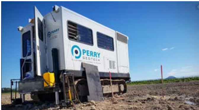
A CPT rig is about the size of a small truck.
