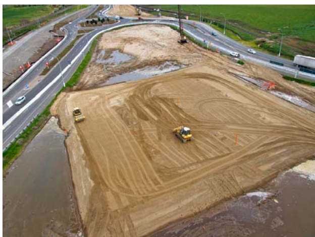
Domain Road trial embankment
