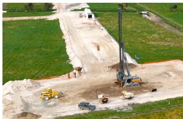
Stone column operation on the Kaituna River east side—early August 2011
