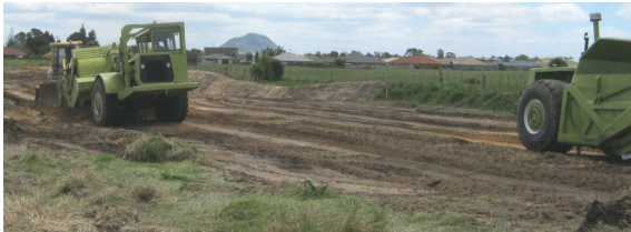
Moterscrapers stripping topsoil
