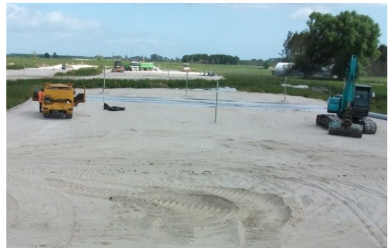
Foundation fill works Pah Road
