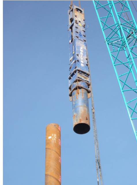
The 9 tonne hammer being lifted into position
