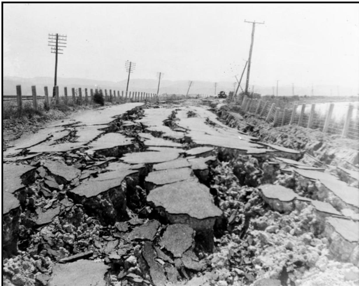
**Figure 2.6: Damage to road from liquefaction and lateral spreading during the 1931 Napier earthquake**
