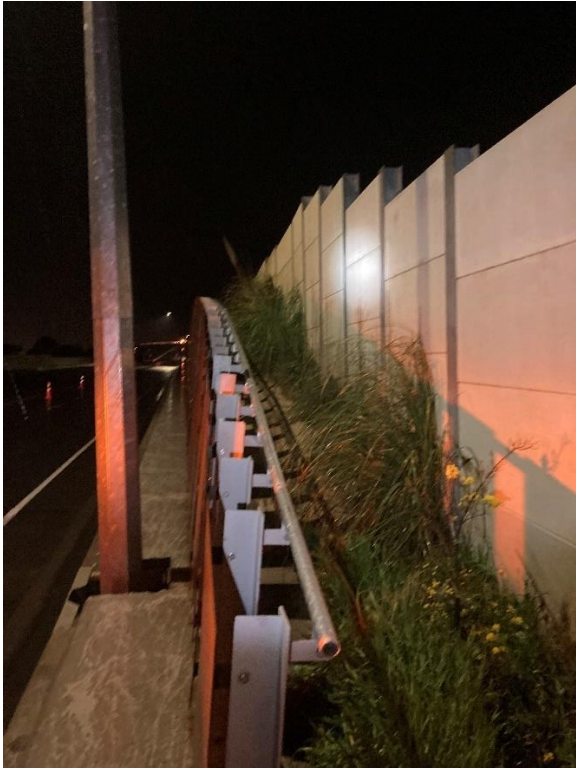
Figure 5 Typical picture of noise wall N3
