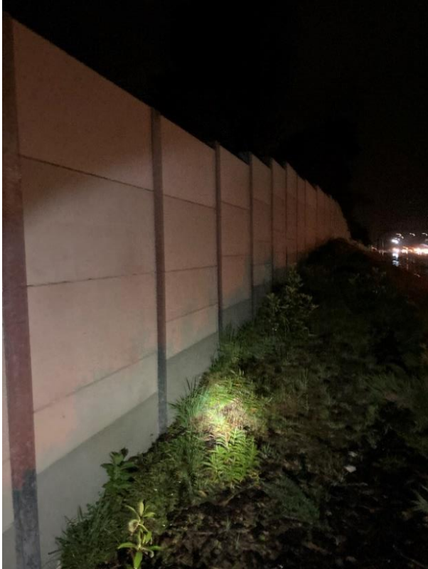
Figure 1 Typical picture of noise wall N4
