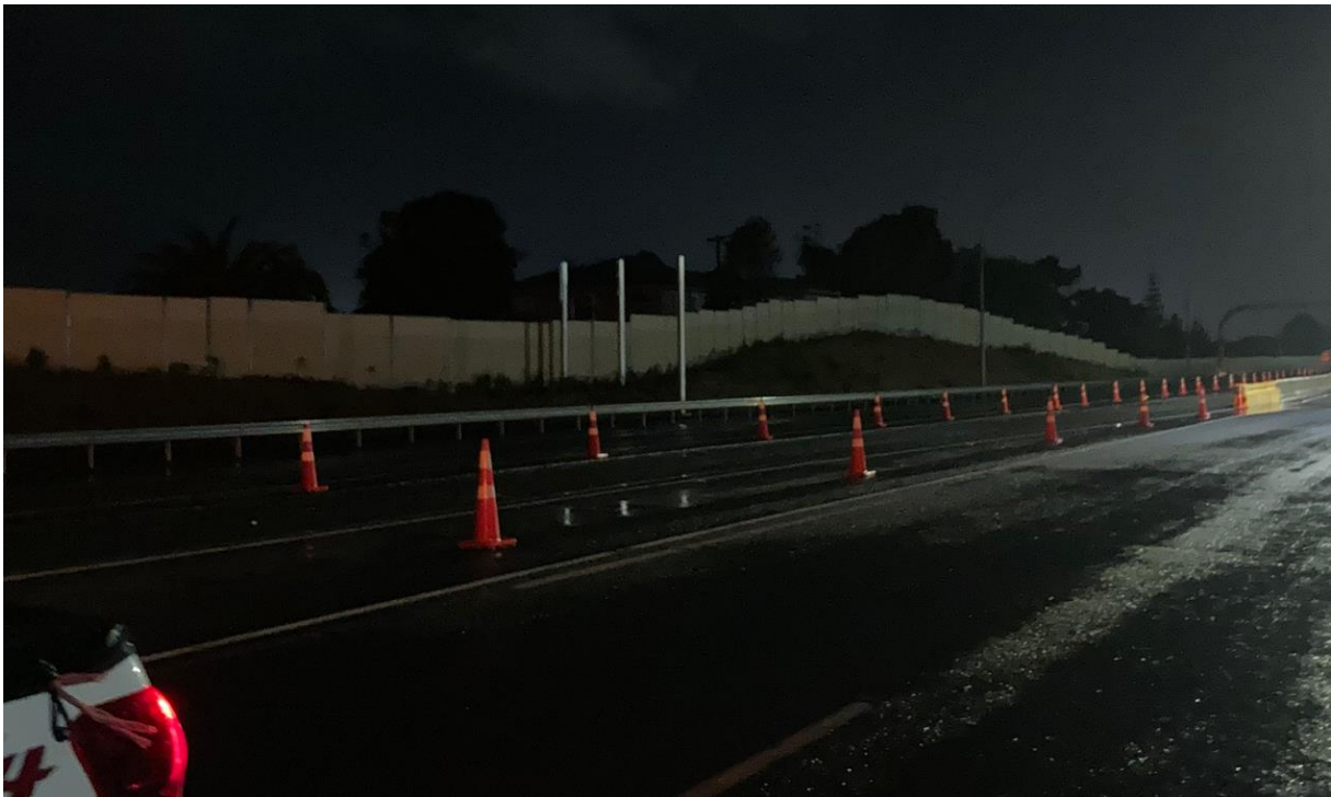
Figure 4 Image of noise wall N4 from site inspection
