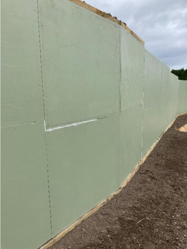
Figure 12 Typical picture of noise wall N2A
