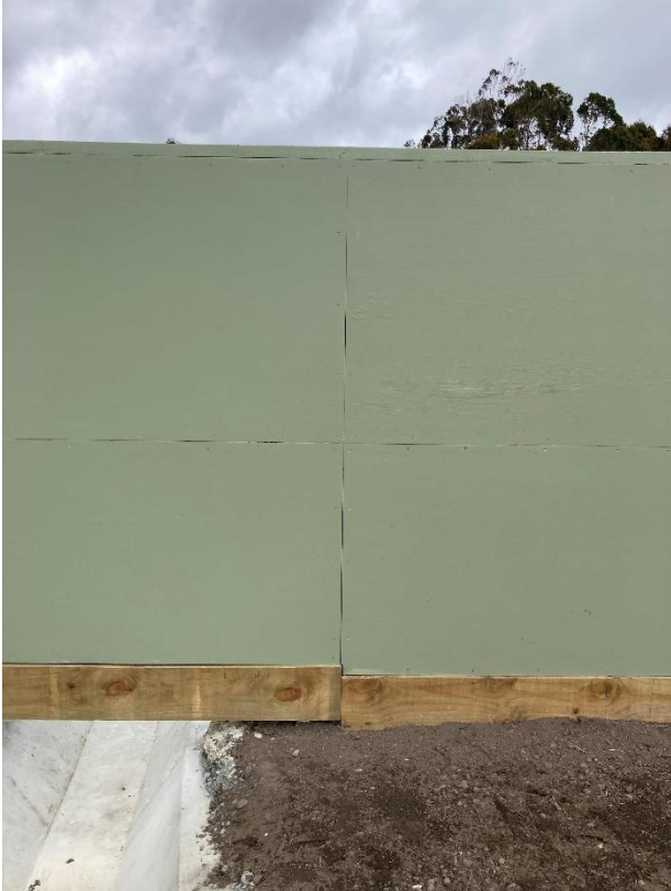
Figure 13 Picture of culvert under noise wall N2A
