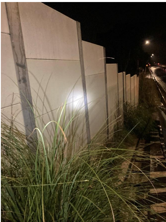
Figure 6 Typical picture of noise wall N3
