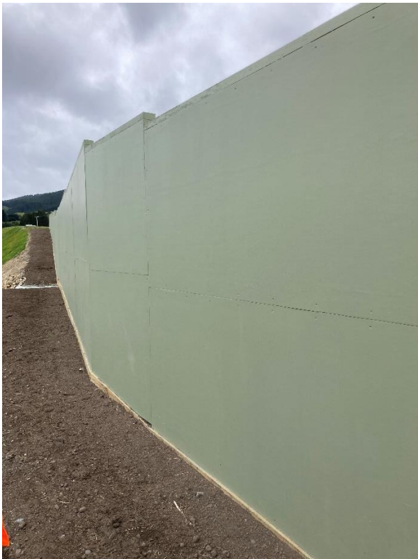
Figure 11 Typical picture of noise wall N2A
