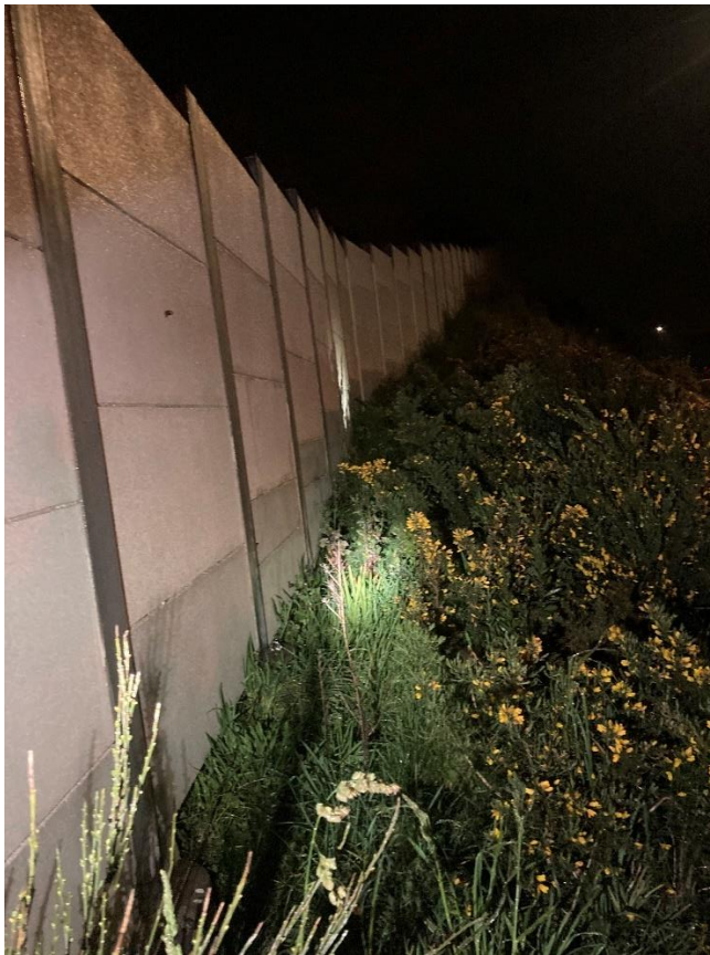
Figure 7 Typical picture of noise wall N2
