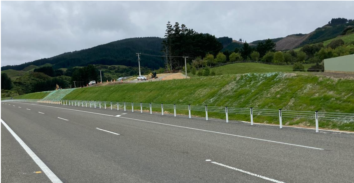
Figure 14 Picture of bund B1/N1A from site inspection
