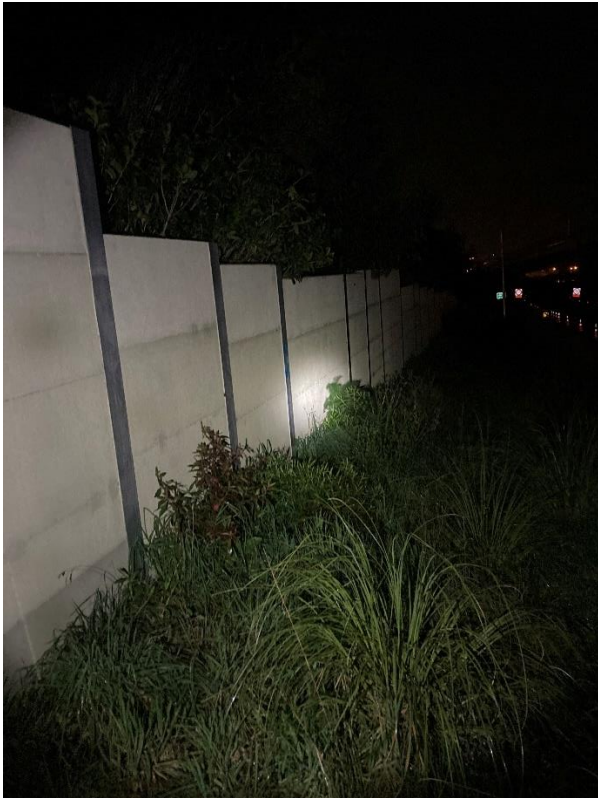
Figure 9 Typical picture of noise wall N6
