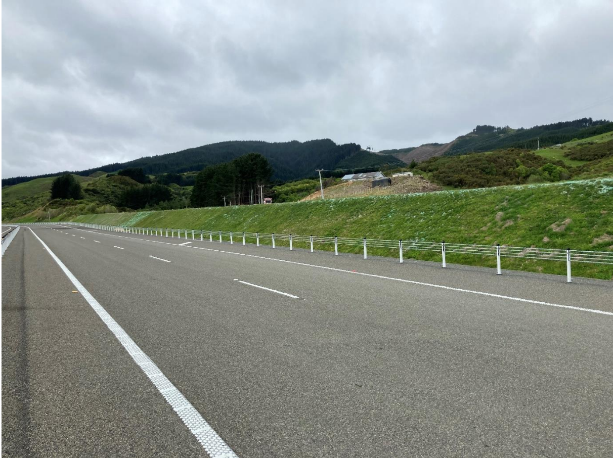
Figure 16 Extent of bund B1 covering location of previous noise wall N1A
