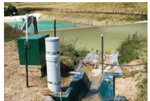
Above: Auto sampling equipment collects water samples from the inlet of the pond, it's then analysed for sediment content.
