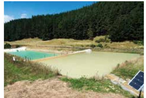
**Above:** Dirty water makes its way into the sediment-retention pond's first bay, where a coagulant is added to help settle sediment out of the water.
