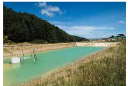
Above: Water then makes its way into the second pond, where sediment continues to settle before water is released into local gullies and streams.
