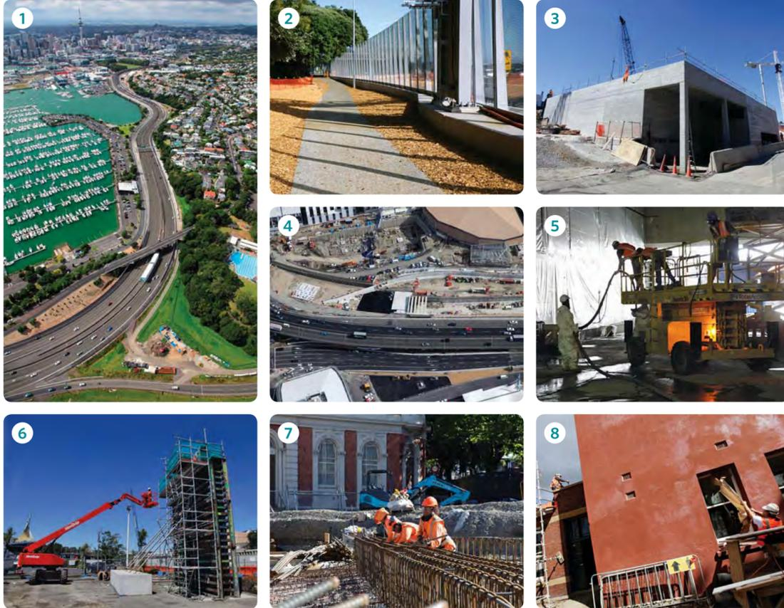
**1. Victoria Park Tunnel:** construction began within Victoria Park in the first week of April 2010 - a year ago. Now: all tunnel walls are completed, the roof is on, 80% of the tunnel excavation is complete and over half of the 54 floor slabs are poured. Interior fit out is underway.
