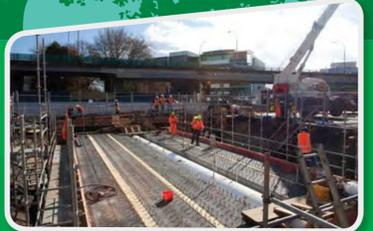
The roof beams are installed between the walls, to hold them in place.
