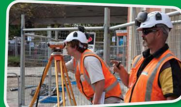
Surveyors mark out the route the tunnel will take and, in particular, the lines the tunnel walls will take.
