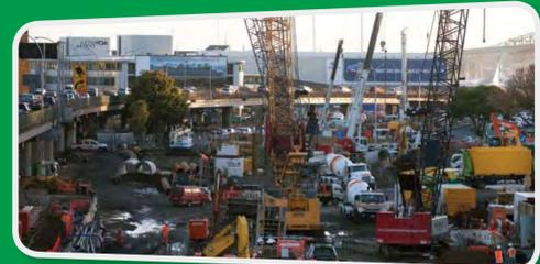
Drilling rigs, cranes and excavators arrive on site and build the walls of the tunnel. There are two ways the walls are being built:
