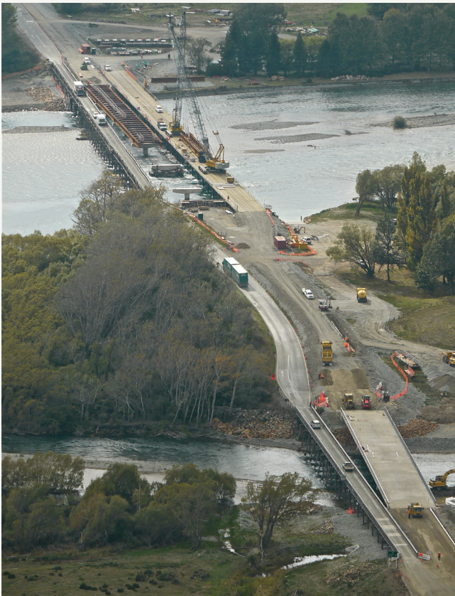
The completed Kurow No. 2 Bridge looking from Kurow toward the river island.
