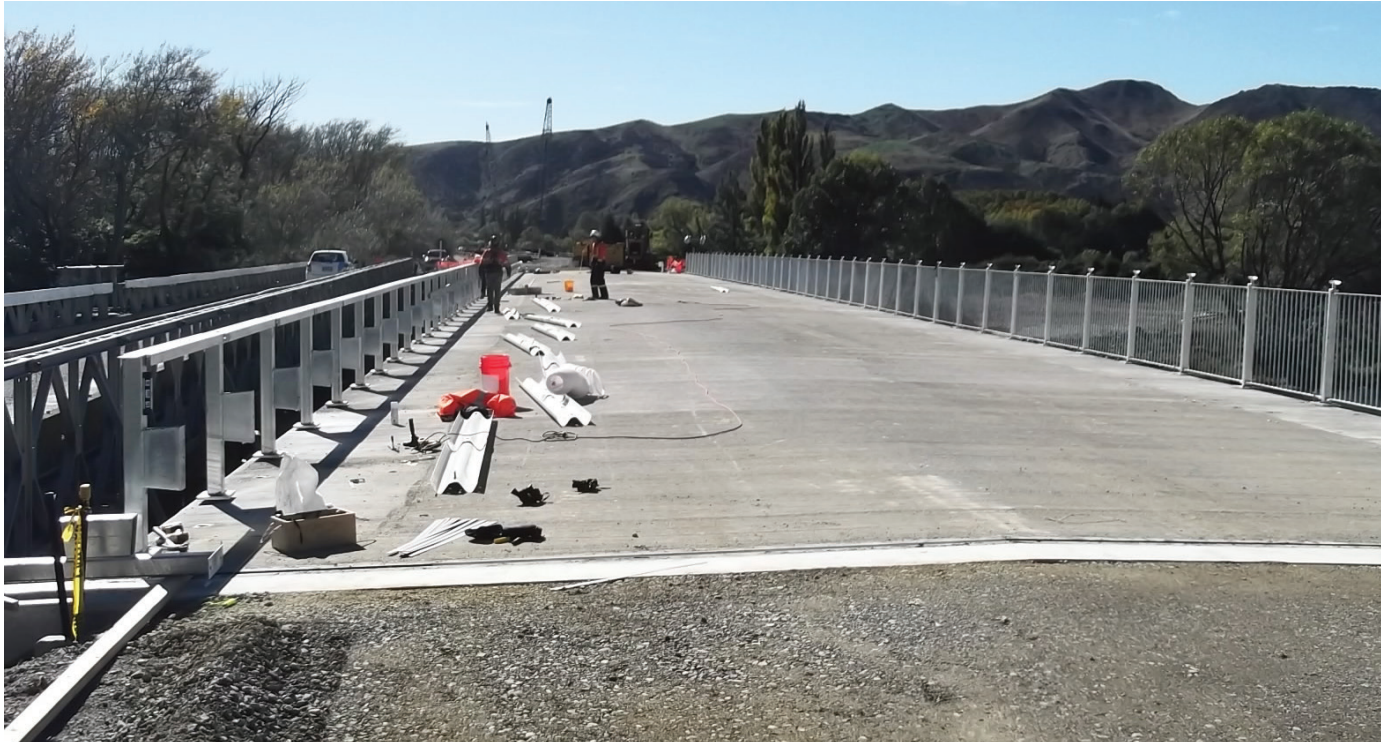
The concrete deck for the new No 2 Bridge.
