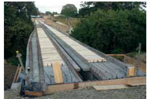
Alford Street Bridge beams are now in place over Te Auaunga.
