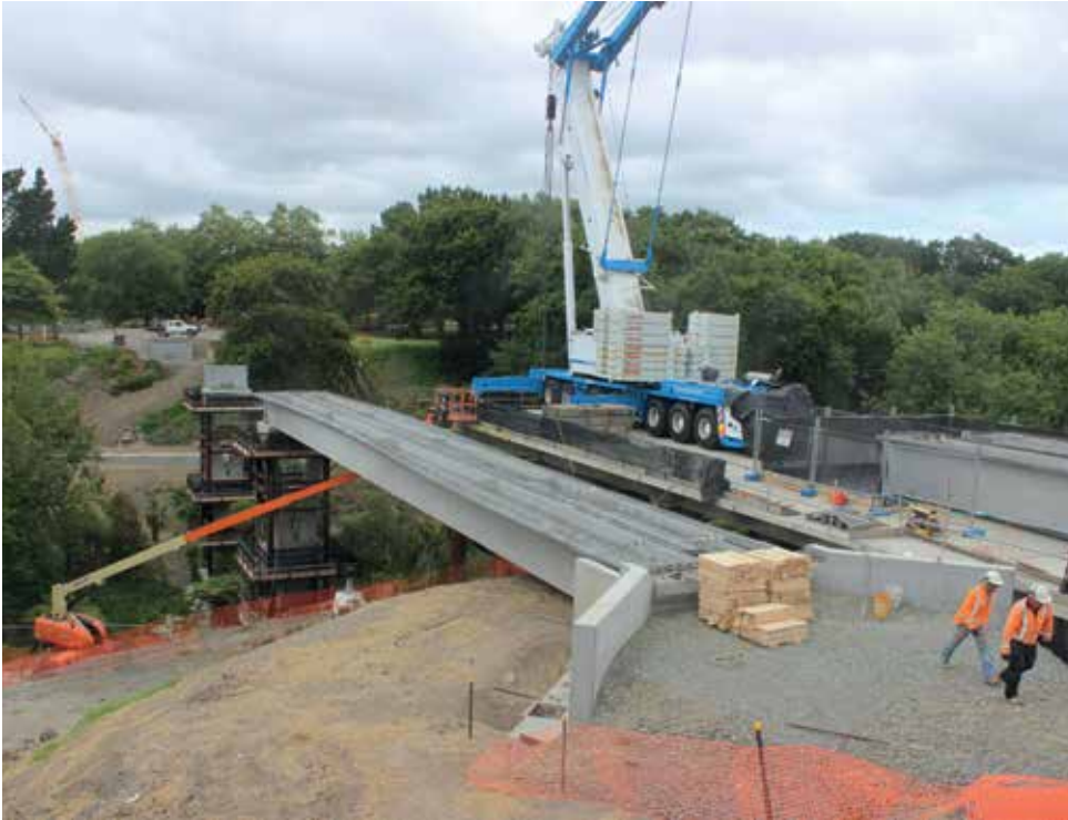
Alford Street is a 90 metre long, 16 metre high concrete footbridge for cyclists and walkers.
