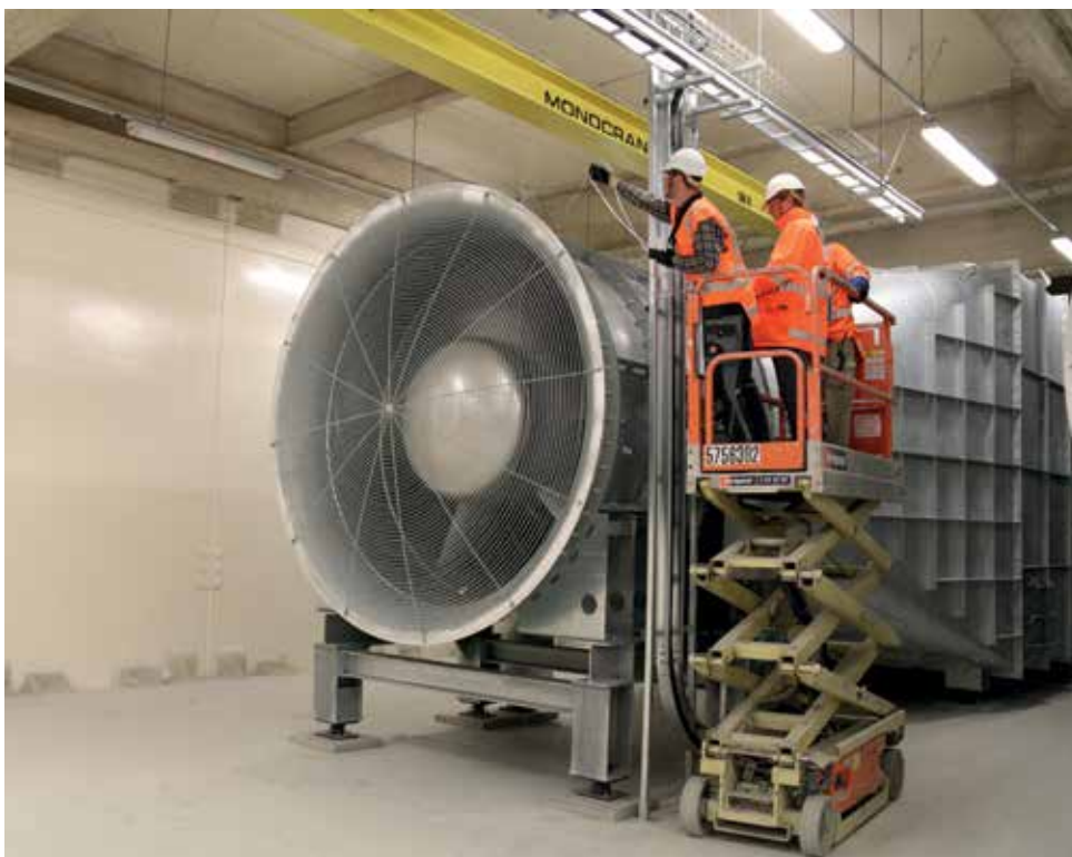
Exhaust fan air flow testing by the Witt & Sohn field engineer.
