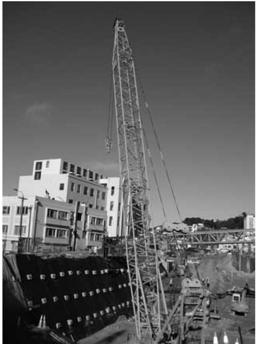
**FULL DEPTH:** An 80-tonne crane at the trench site off upper Willis Street, where excavation in the first section has reached the full depth of eight metres. The concrete blocks in the photo are attached to temporary soil nails inserted into drilled holes and grouted into place. These steel nails are 4-14 metres in length and support the cut slopes while the first section of the 150-metre concrete trough is constructed.
