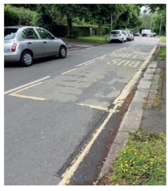
The cohesive strength of the substrate, at various temperatures, must meet or exceed the expected traffic loadings (to prevent cohesive substrate failure).
