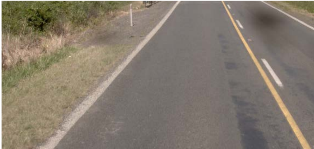
Figure C.16 3% in- situ stabilisation – SH26-RS80-13577-13584 (decreasing side) – 16- month inspection
