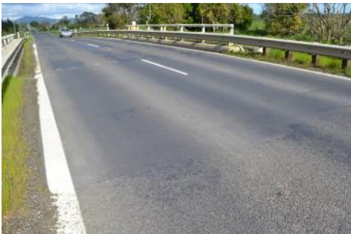
Figure C.25 Mill and AC inlay – SH26–RS80–13596–13606 (decreasing side) – 3- month inspection
