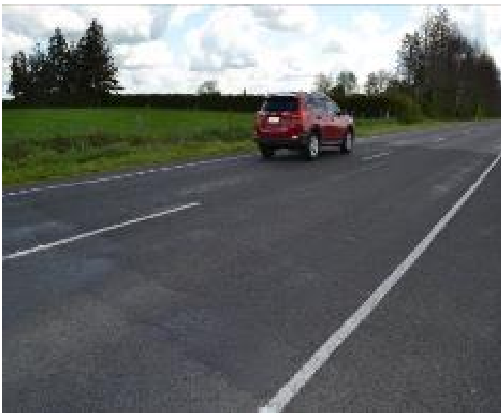
Figure C.28 3% in- situ stabilisation – SH27–RS46–17982–18012 (decreasing side) – 3- month inspection
