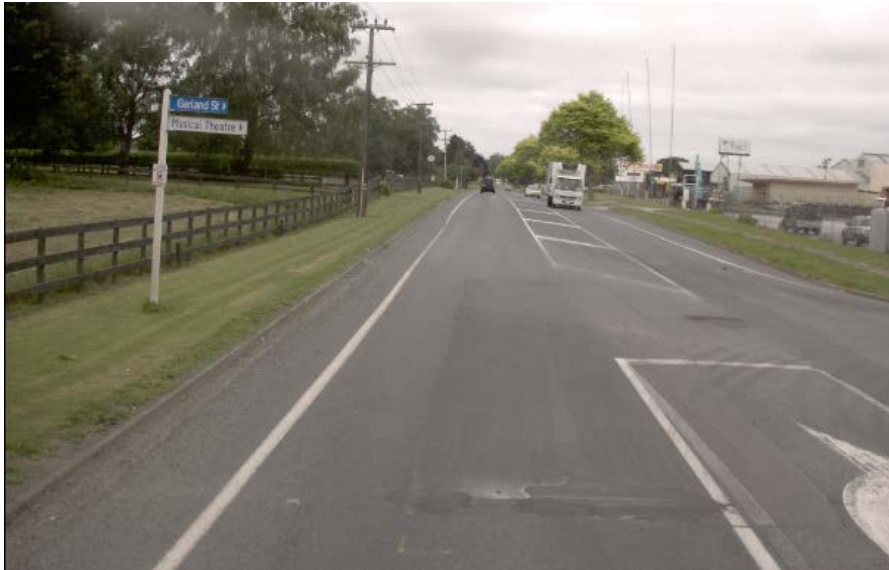
Figure C.12 Mill and AC patch - SH24-RS0-1975-1994 - 16- month inspection
