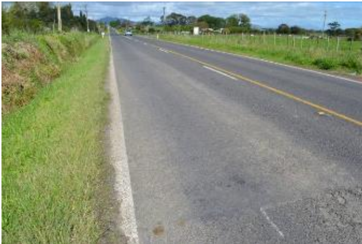
Figure C.18 1.5% in- situ stabilisation - SH26-RS80-13304-13364 (decreasing side) - 3- month inspection
