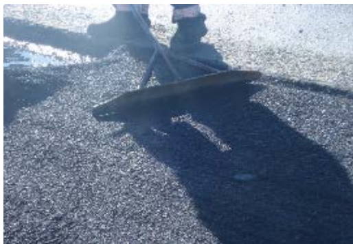
Spread asphalt using a bob-cat with a spreader.
