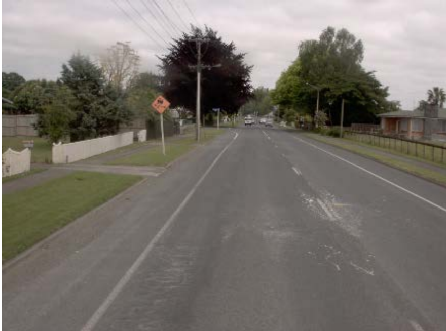
Figure C.3 3% in- situ stabilisation - SH24-R50-1417-1440 - 16- month inspection
