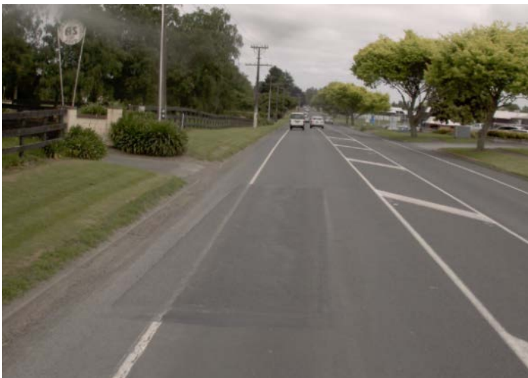
Figure C.9 Full depth granular reconstruction – SH24-RS0-1975-1994 – 16- month inspection
