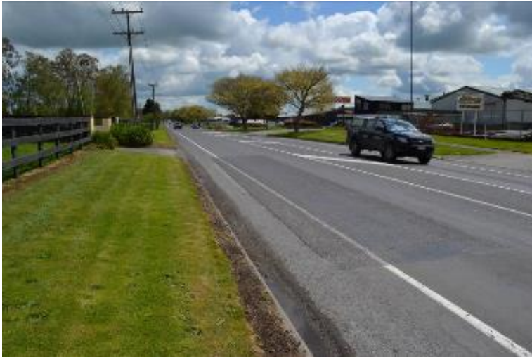
Figure C.8 Full depth granular reconstruction – SH24-RS0-1975-1994-3- month inspection
