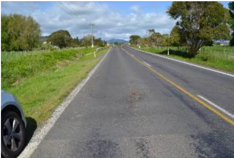
Figure C.14 3% in- situ stabilisation – SH26–RS80–13577–13584 (decreasing side) – 3- month inspection
