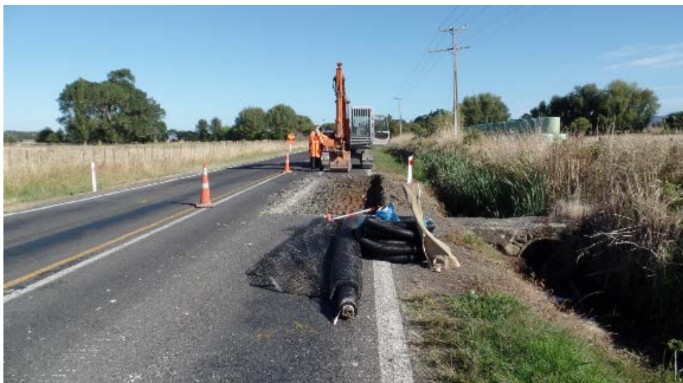
Figure C.21 Full depth granular reconstruction – SH26-RS80-13394-13434 (decreasing side) – construction
