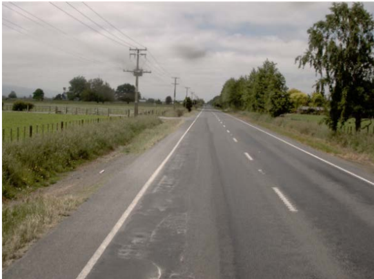
Figure C.32 1.5% in- situ stabilisation – SH27-RS46-17430-17466 (decreasing side) – 16- month inspection
