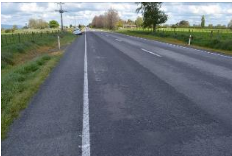
Figure C.31 – 1.5% in- situ stabilisation – SH27-RS46-17430-17466 (decreasing side) – 3 month inspection
