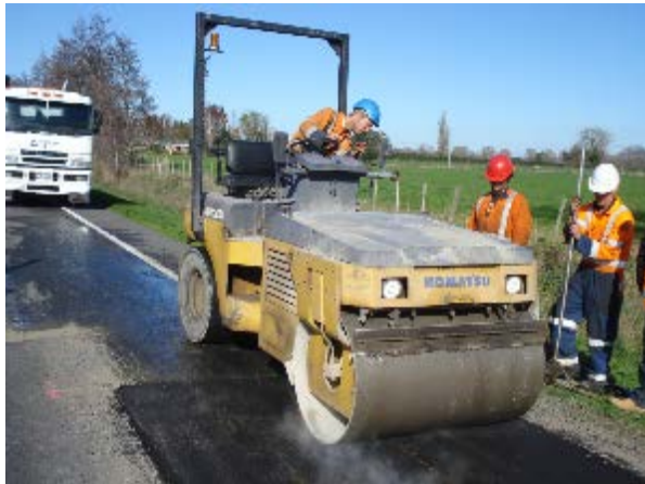
Four to six passes to compact asphalt layer.
