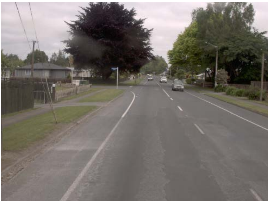
Figure C.3 3% in- situ stabilisation - SH24-R50-1417-1440 - 16- month inspection
