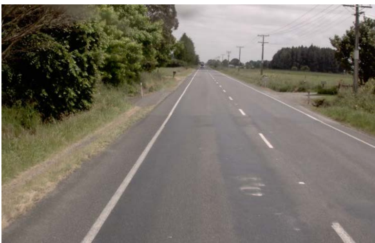
Figure C.29 3% in- situ stabilisation – SH27–RS46–17982–18012 (decreasing side) – 16- month inspection
