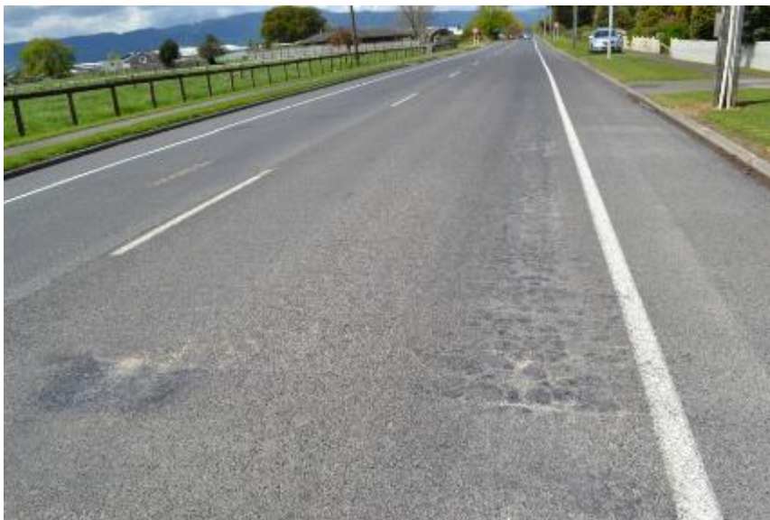
Figure C.1 3% in-situ stabilisation – SH24–RS0–1417–1440 – three month inspection
