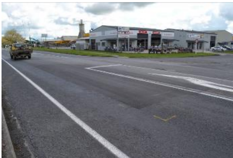
Figure C.11 Mill and AC inlay – SH24-RS0-2093-2112 – 3- month inspection
