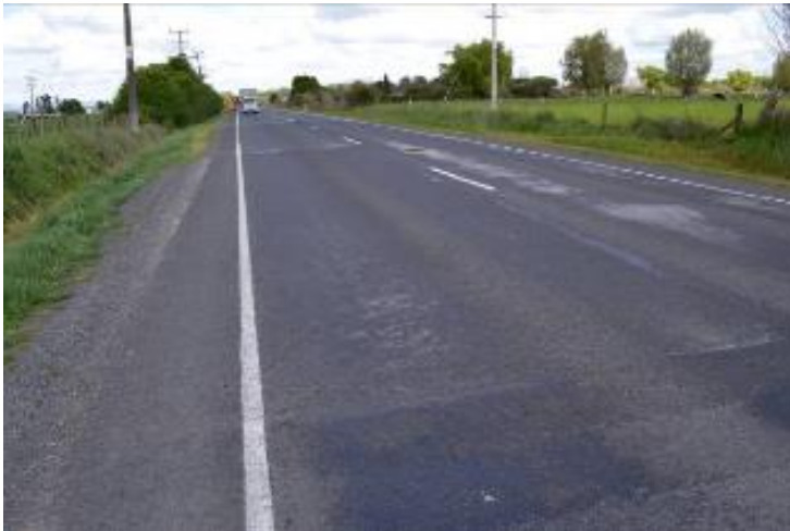
Figure C.34 – Full depth granular reconstruction – SH27-RS46-17965-17980 (increasing side) – 3- month inspection
