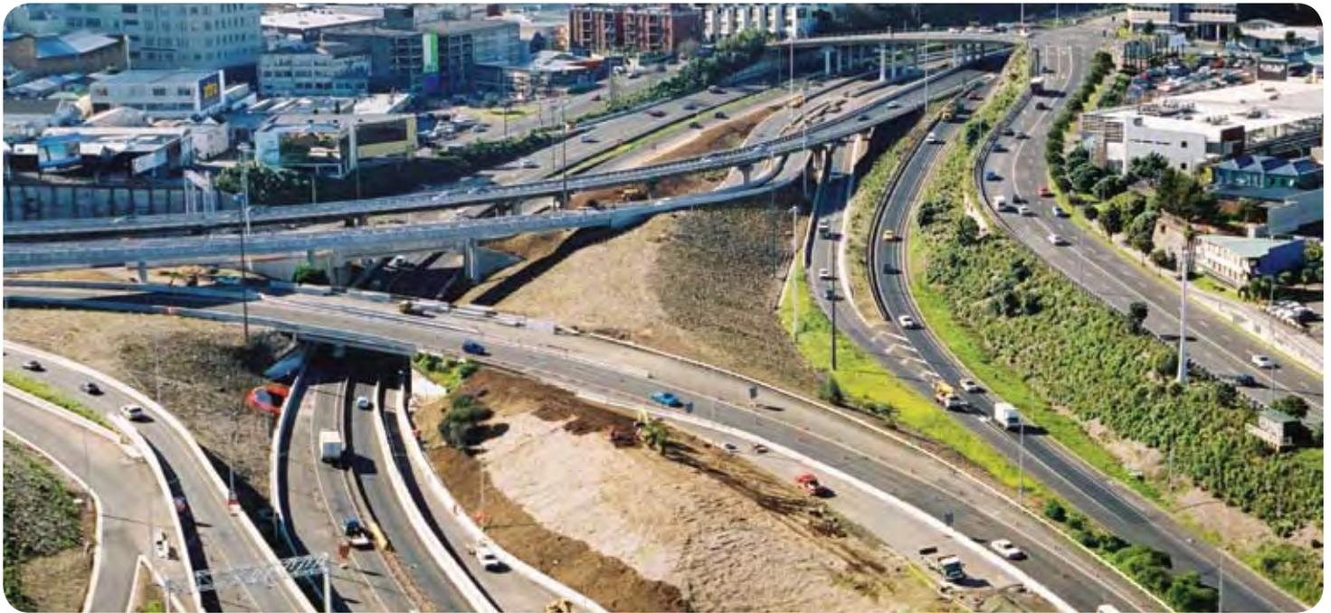
Construction of the multi-million dollar project started in January 2004, comprising the four new links between SH1 and SH16, two new off-ramps to Nelson Street from the Southern and Northwestern Motorways, and new lane layouts to make the motorway safer and more intuitive to use.
