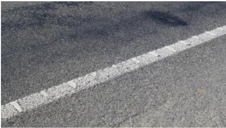
Figure 6-3: ATPM loss due to snow ploughing (from Lester et al (2017))
