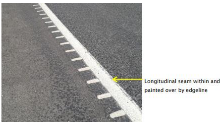
Figure 11-1: A well carried out in-lane reseal (Lester et al 2017, page 14)
