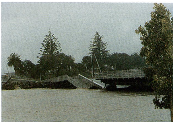
Figure 10.5: Wairoa Bridge failure (1988). This bridge failed following scour of the bed which was exacerbated by debris.
