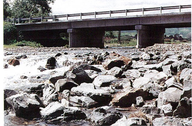
Figure 10.10: Riprap weir below the Waikanae River Bridge
