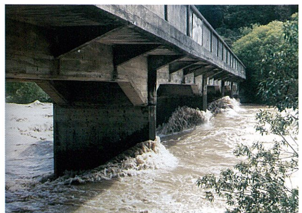
Figure 10.7: The effect of piers on the flow of a river in flood.
