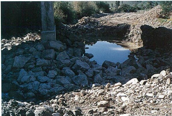
Figure 10.9: Wai-iti Bridge – protection against local scour.
