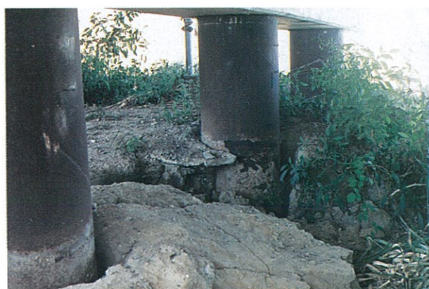
Figure 11.3: Movement of piles in the ground.
