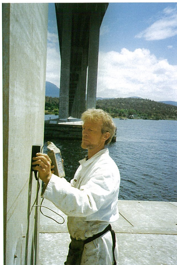
Figure 3.7: Detection of reinforcing steel using an electromagnetic covermeter
