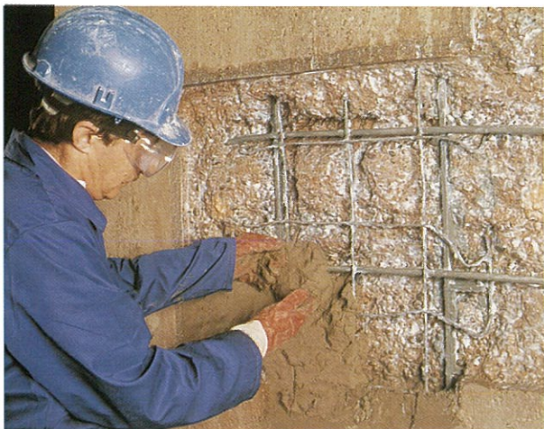
Figure 3.9: Initial application (by hand) of a trowellable mortar.
