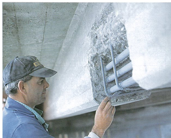
Figure 3.12: Prepared excavation showing sawcut edges and application of reinforcement primer.
