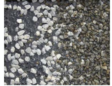
Application of the second chip
