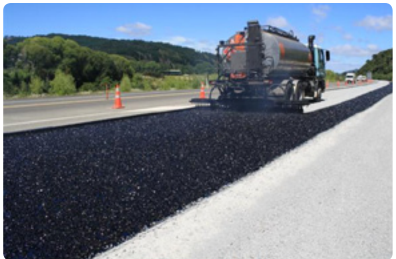
Widening of SH2 at Silverstream (Wellington)
