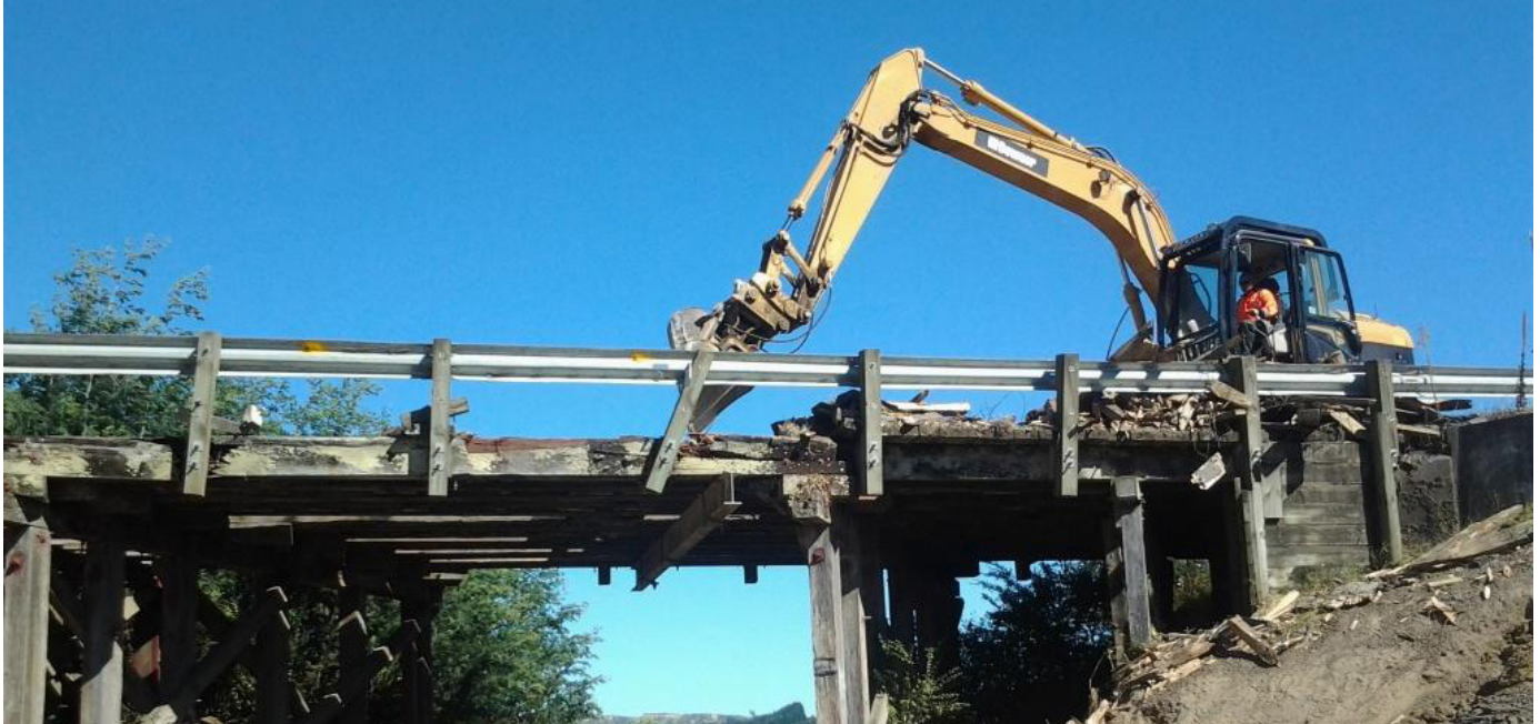
Taneatua rail overbridge
