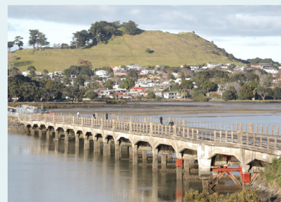
Old Māngere Bridge, SH20, Auckland
