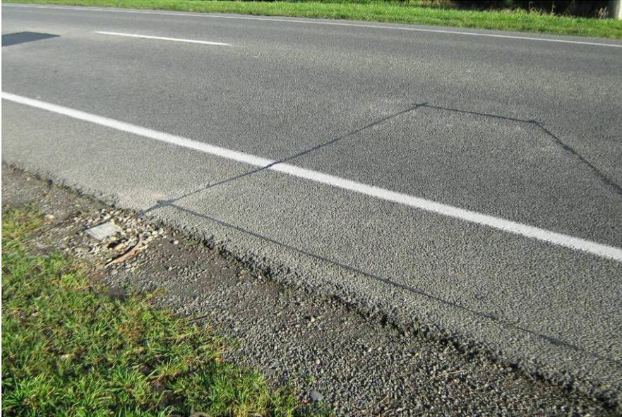
**Figure 20: Sparks Road trial site –Bicycle Recorder loop**
