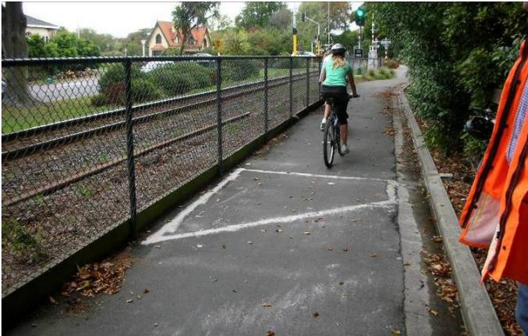
*Figure 12: Bicycle recorder loop on the railway cycleway*
