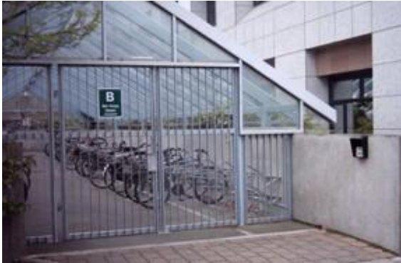
Figure 29: enclosure with swipe card access, electric gate, security cameras – Univ. of Canterbury (G. Koorey)
