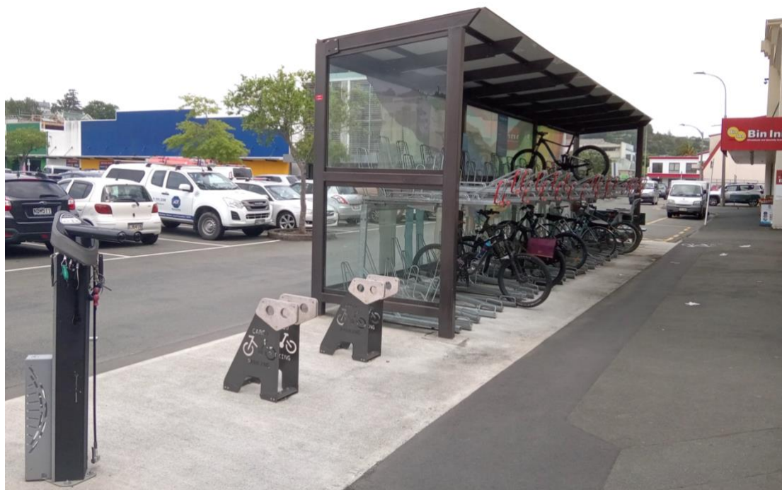
Figure 22: double-tier shelter with cargo stands and tool stand in foreground, Nelson (M. Edwards)
