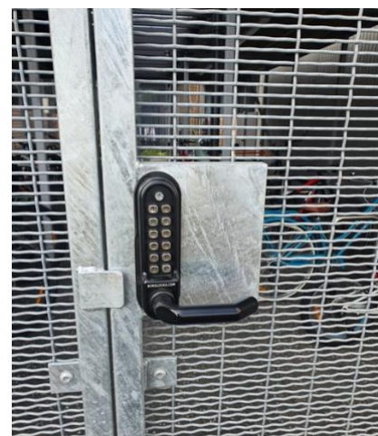
Figure 36: galvanised steel mesh and frame; pushbutton lock (A. Heins)
