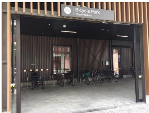
Figure 31: cycle parking with motorised sliding doors and e-bike charging, Christchurch bus exchange (J. Lieswyn)
