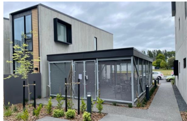
Figure 34: a bike enclosure in the East Frame residential development, Christchurch (J Lieswyn)
