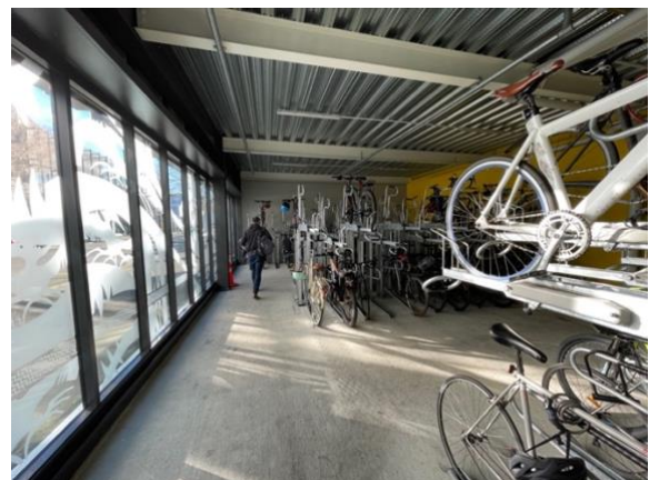
Figure 32: access-controlled public bike parking in a parking building, Christchurch (J. Lieswyn)
