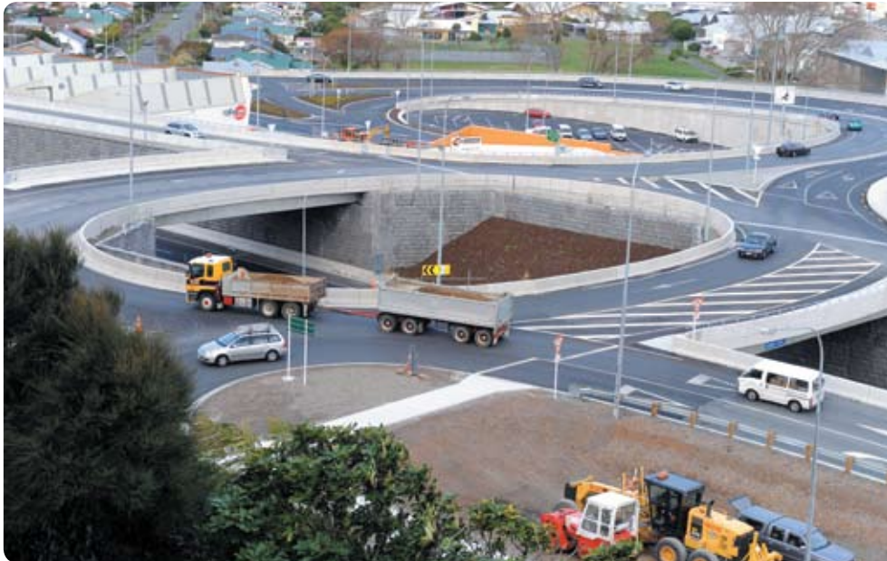
Construction of Dowse Interchange on State Highway 2 in Lower Hutt.
