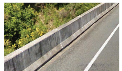
c) Rigid concrete barrier (segmental system)
